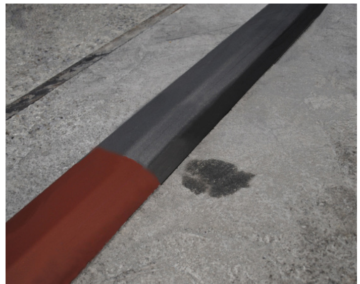
Fig 3. Use of an anti-galvanizing paint solution as a masking system
