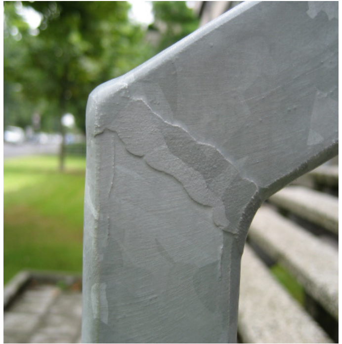
Fig 4. A weld that was ground flush prior to galvanizing. The high silicon content of the weld metal has then led to a thicker coating forming locally
